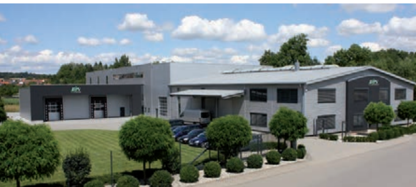
2008 – Triplication of the plant area
